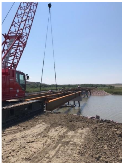
Setting beams at Lower Brule
