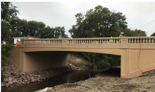
Nearly completed bridge in Yankton, SD
